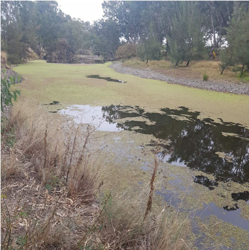
Photo 3. Wells Crossing at Three Mile Bridge showing an accumulation of reeds because the water isn't flowing in order to clear it out.
